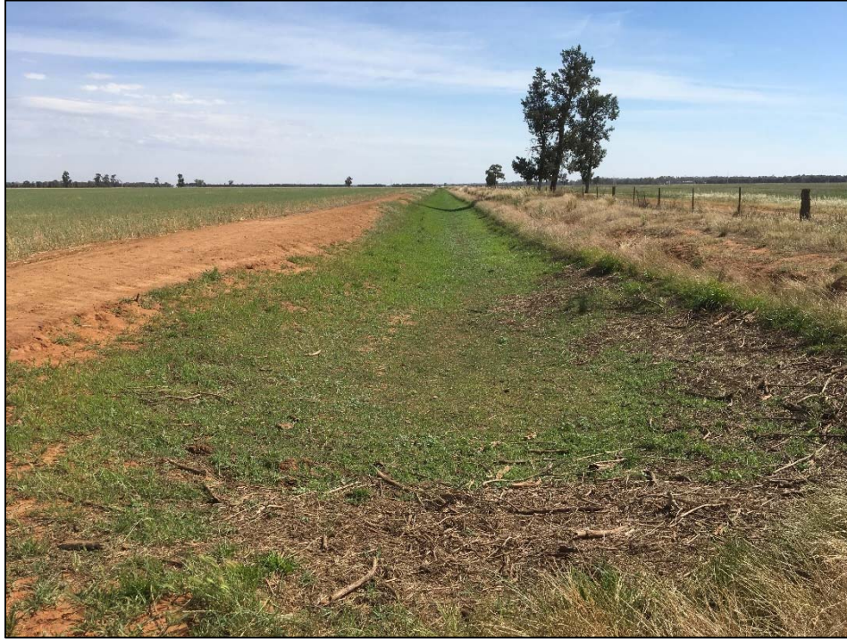
Figure 3-4 Unnamed irrigation channel
