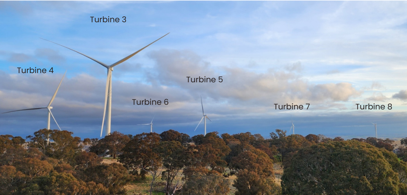
Collector Group 3 turbines constructed to date at the Flyers Creek Wind Farm
