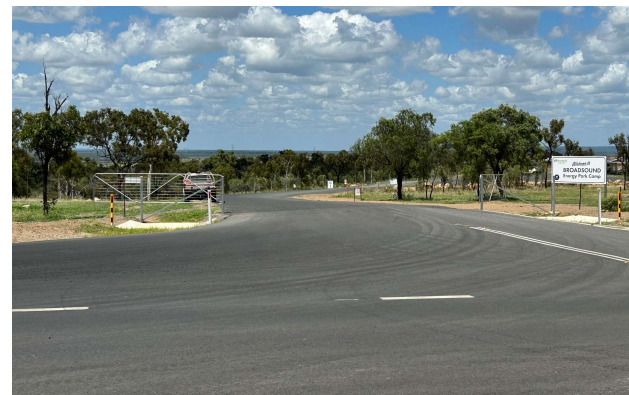
Completed Site Entrance
