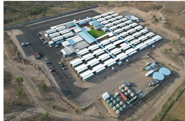
Broadsound Solar Farm Construction Camp
