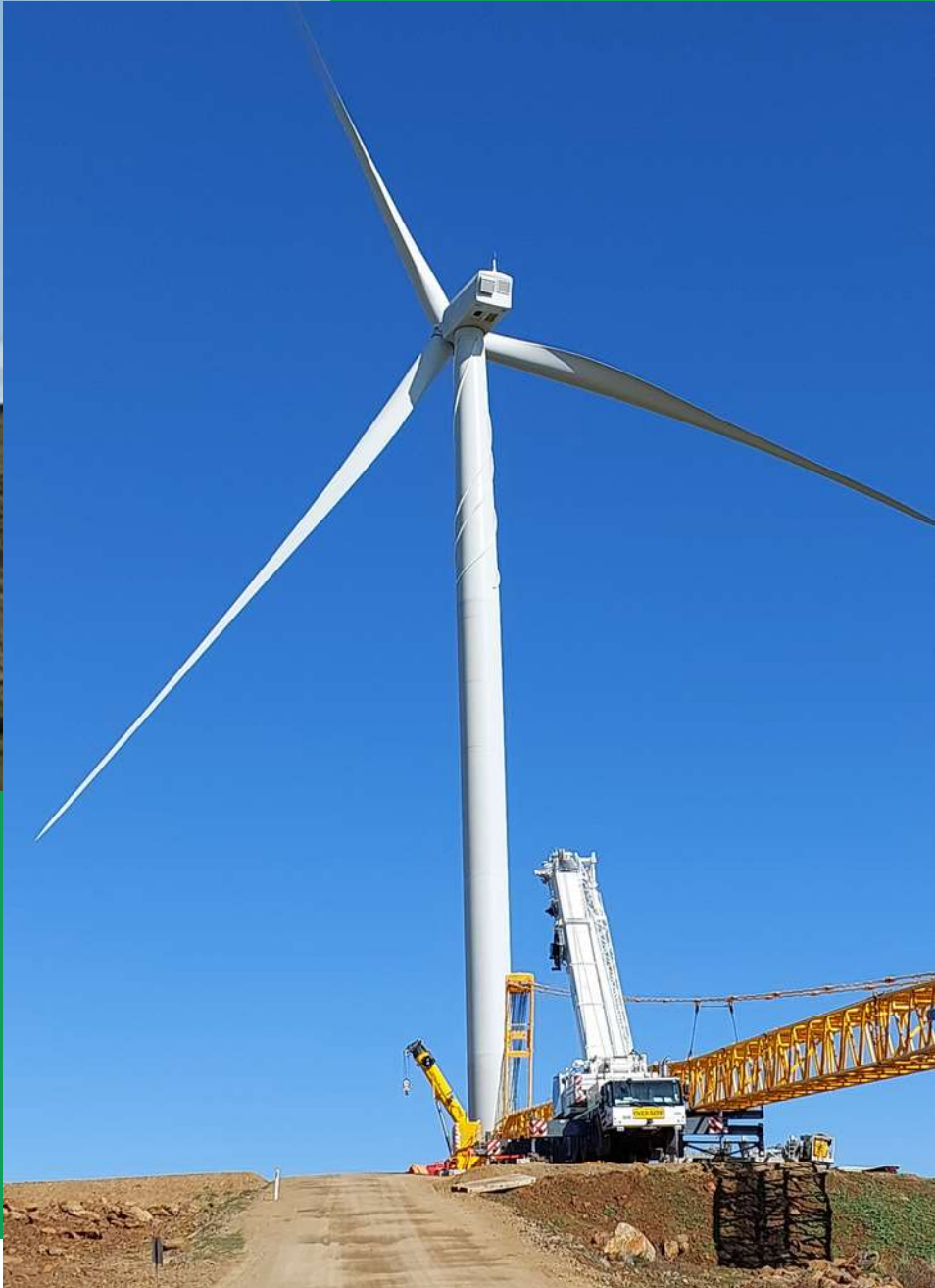
Turbine 19, three blades installed Collector Group 2-West 2 August, 2023
