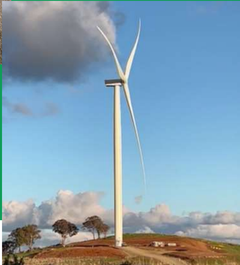
Blades of Turbine 7 in Collector Group 3 turning to export the first electricity from Flyers Creek 31 August, 2023
